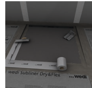
Seal the joints between the wedi Fundo shower element and adjacent surfaces with the wedi Fundo sealing set.
